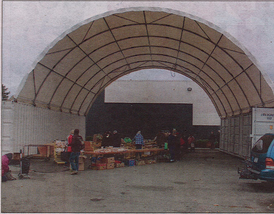
The Fraser Valley Regional Food Bank recently added a massive tented area stretched up and between two shipping canisters in order to continue to serve people outside during the winter. The need for the food bank continues to increase, says director Matthew Campbell. (Photo: Malin Jordan)
